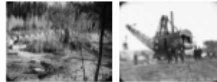
Fig. 4 a,b. Attempts were made to control flooding of the river. Fig. 4a. Left, taken Dec 26, 1915 shows dam barriers. Fig. 4b. Right, Dredge excavator used at the reservation cutoff, Oct 23, 1915. Photos courtesy of the Washington State Historical Society, Puyallup River Rechanneling #17 and #22.
